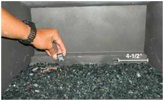
Log bracket install
