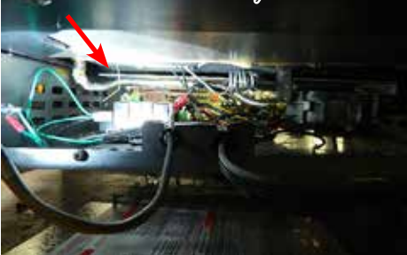
Location of the Aeration Adjustment wire
