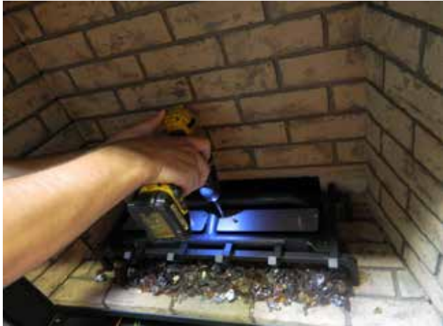
Diagram 5—Install Log support plates
