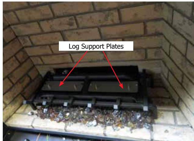
Diagram 6—Log support plates installed
