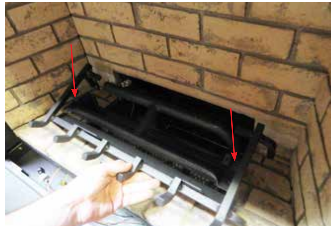
Diagram 2—Log Grate Install
