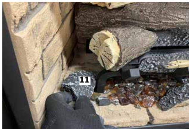
Diagram 16-Install Log 11
