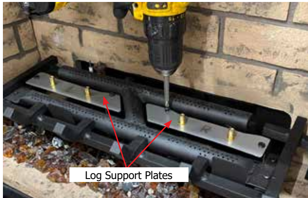
Diagram 5-Install Log support plate installation
