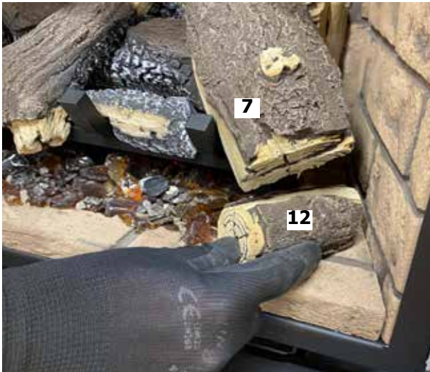
Diagram 17-Install Log 12
