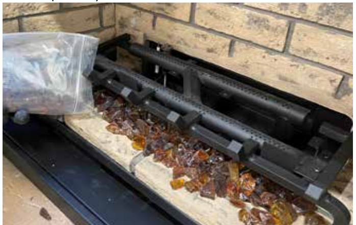
Diagram 3-Install Glass
