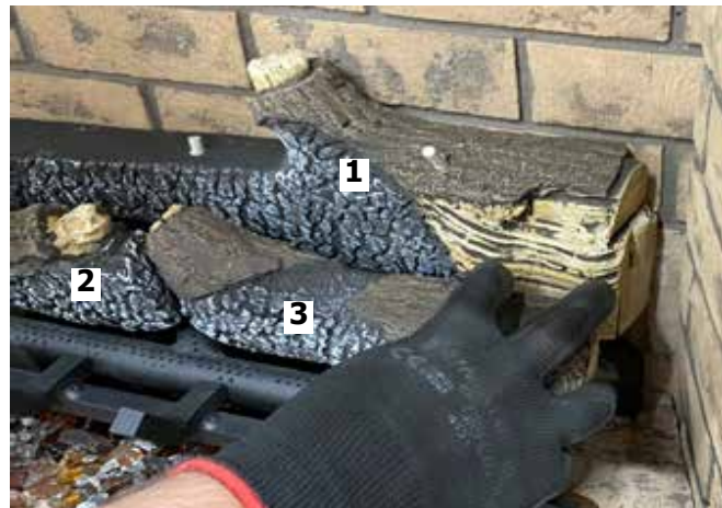
Diagram 8-Install Log 3
