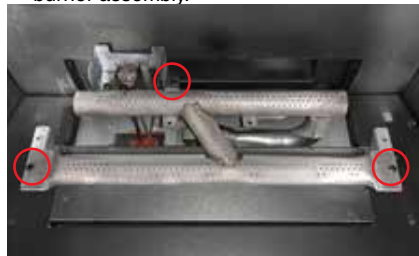
Diagram 2: Slide burner assembly to the right—then remove.
