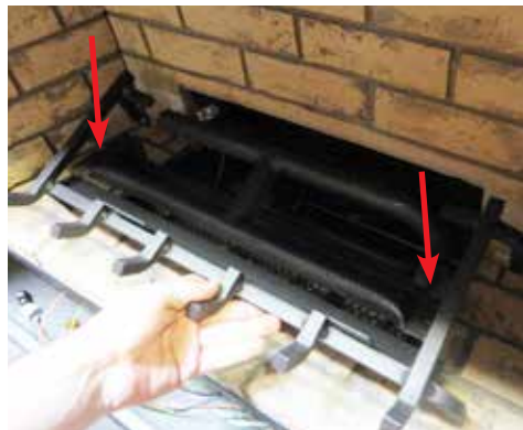
Diagram 1: Remove the left and right screws.
