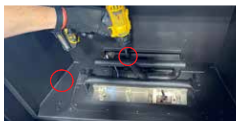
Diagram 2: Slide burner assembly to the right—then remove.
