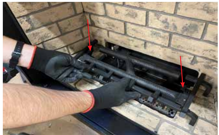
Diagram 2-Log Grate Install
