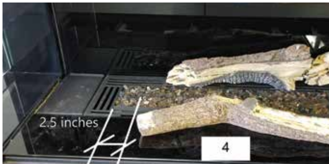
Log 4 to edge of burner
