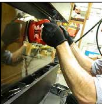
Handle glass with supplied vacuum clamps
