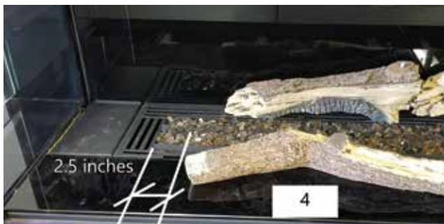
Log 4 to edge of burner
