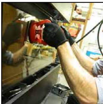
Handle glass with supplied vacuum clamps
