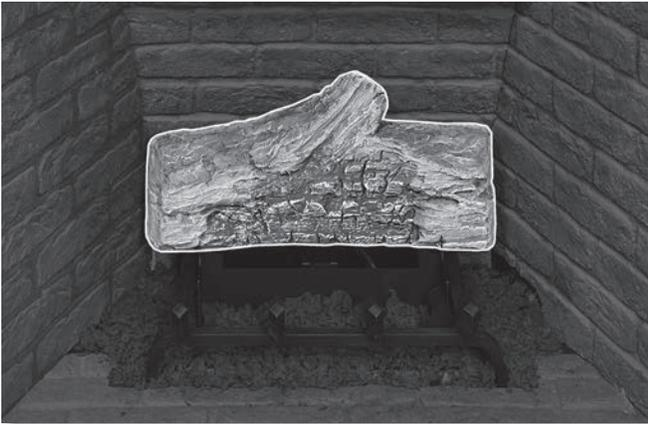
Figure 34: Log Set Installation - Step 1
