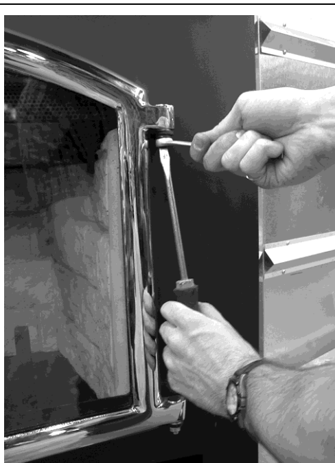
Figure 6 Door Hinge Adjustment
