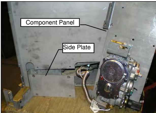
3. Remove Side Plate and knockout if present (see millivolt section). Place Component Panel on other side of valve.
