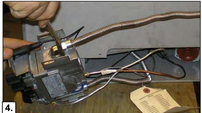
**4.** **Optional-** Connect flex (Not included. Order PN# FP15GC) to inlet side of valve. This can then be connected to the gas supply and routed through the channel inside the fireplace.
