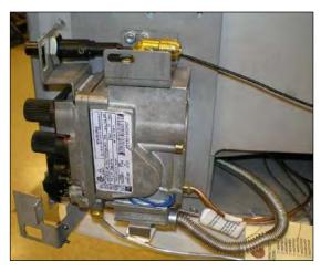
Step 1: Disconnect pilot lines and gas supply line from valve on the side of the unit. NOTE: Care should be taken to ensure that the gas and pilot lines are not damaged during handling. These lines are fragile.
