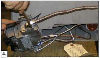
**Optional-** Connect flex (Not included. Order PN# **FP15GC**) to inlet side of valve. This can then be connected to the gas supply and routed through the channel inside the fireplace.
