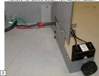
Attach Fan Control Switch Extension Bracket using [2] #6
