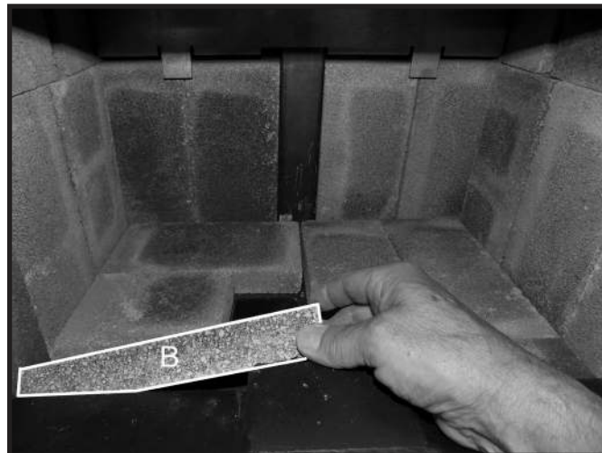
Figure 30: Final narrow brick in place.
