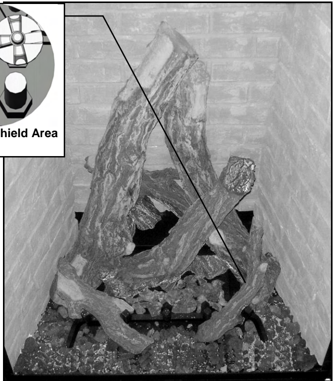
Step 6: Add lava rock to the bottom of the burner pan. Add glowing embers to the top of the ember plates and front burner tube. Sprinkle vermiculite over the lava rock. Do not place any media within Pilot Shield Area (see above).
