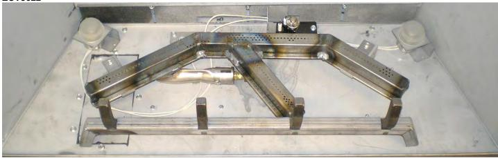
**STEP 3**: Place Lamps in position in firebox. Attach to fireplace with a single screw at the locations shown above for each unit. Lamps can be placed facing upward or sideways. Replace burner tube and false bottom, along with pilot shield.
