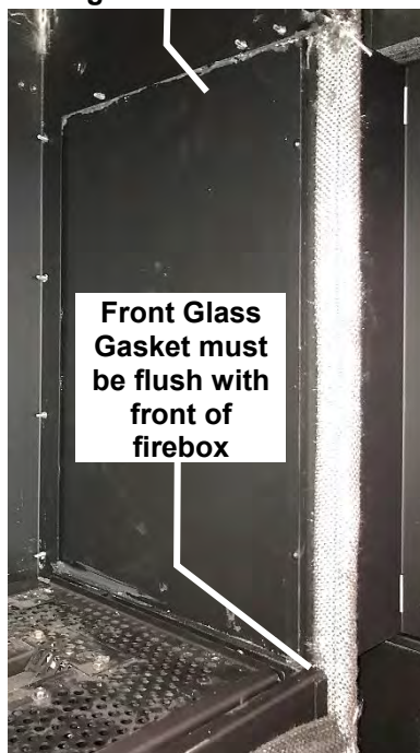
C Ensure Seal Gasket and Mill-Pac are sealed against the side of the firebox
