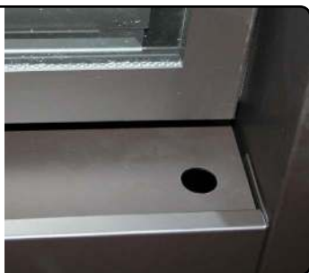
Figure 20.b Removing and installing the Horizontal Access Panel
