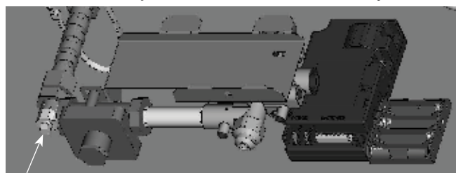
1/8" Inlet line gas pressure 'test point' plug (in control compartment)
