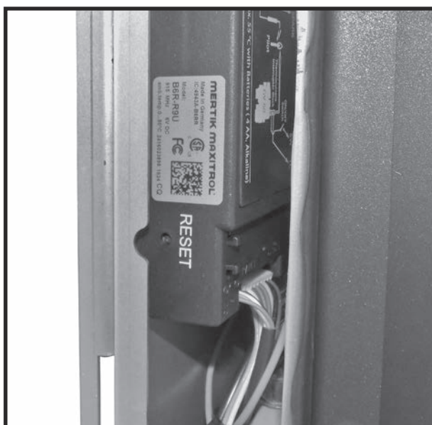
Figure 95: Maxitrol reset button location.
