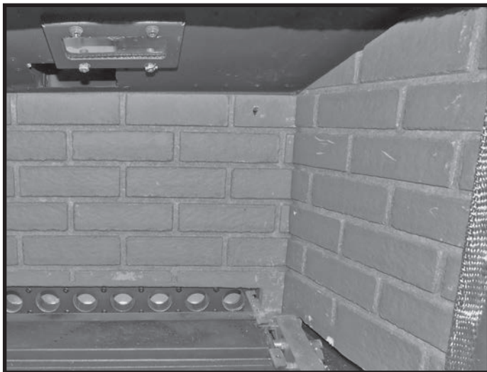
Figure 27: Right side panel in place.
