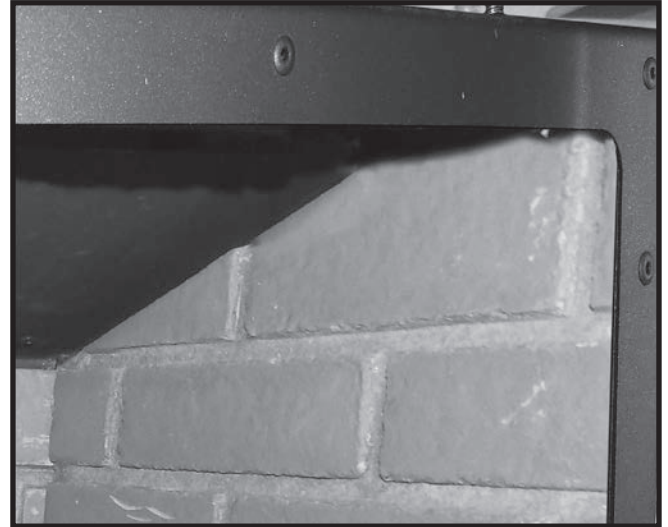
Figure 26: Upper firebox corner and gasket.
