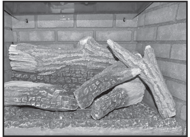
Figure 81: 5th log placement.
