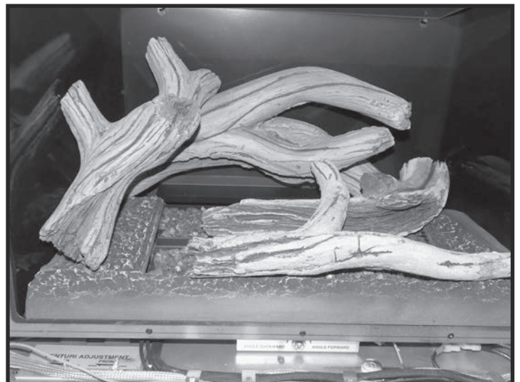
Figure 98: Fourth log placement.
