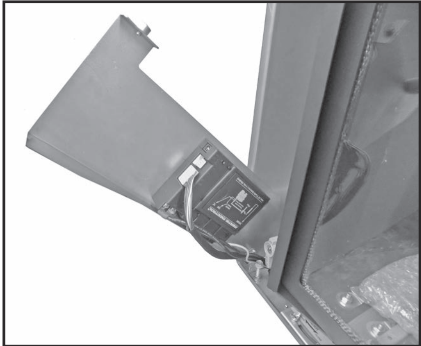
Figure 40: Maxitrol electrical controller in its caddy.
