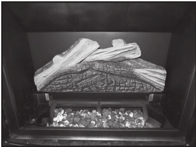
Figure 46: Number 1 log set in place.
