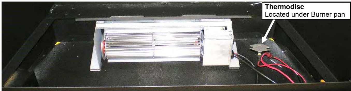
Fan installed in fireplace. Burner removed for clarity.
