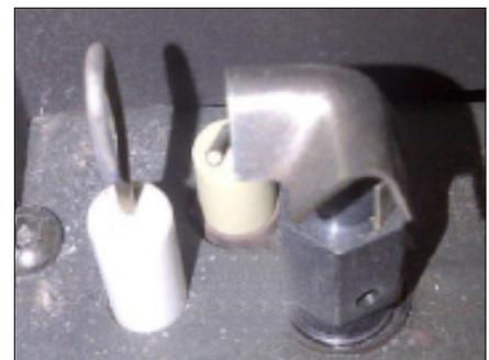
Figure 20: Proper Pilot Position
