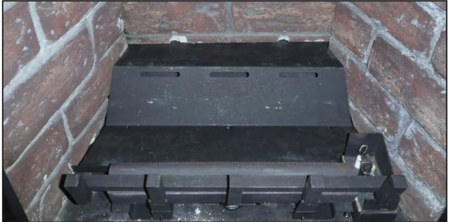
Figure 41. Empty firebox with grate and locator pins.
