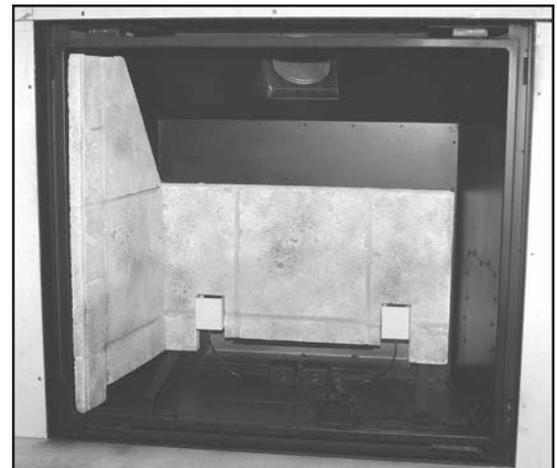
**Figure 64: Left Firebox Liner Panel in Place.**
